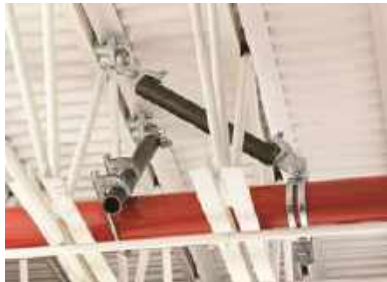
BAR JOIST ATTACHMENT
